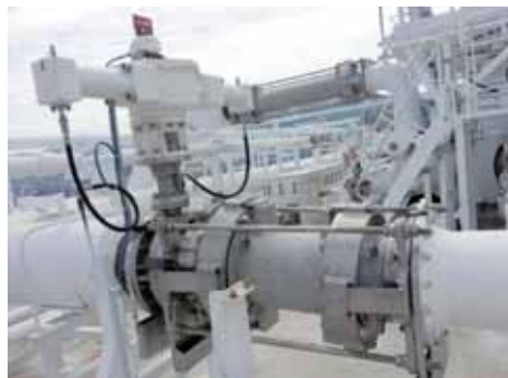
Installation on the ship
