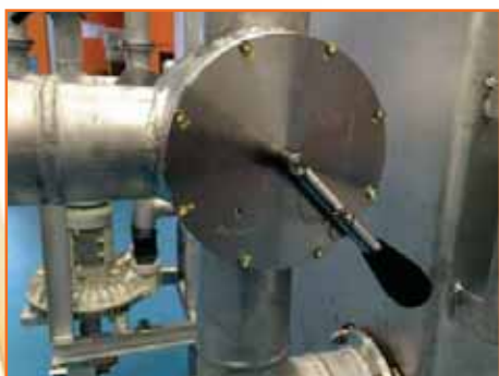
Detail of three-way valve for maintenance
